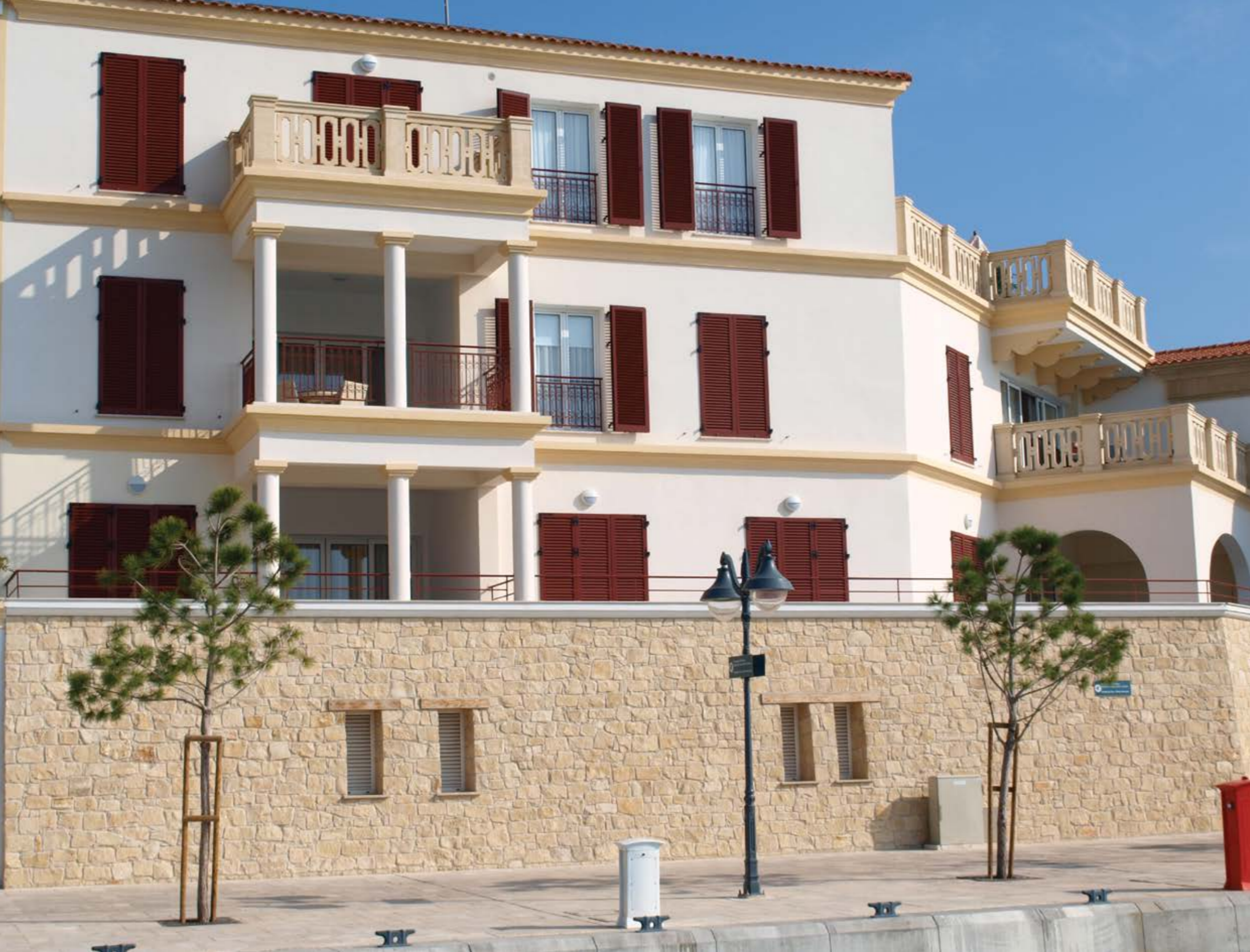
Project: Thetis Residences, Limassol Marina Architects: Atelier Xavier Bohl (France) Material application: Wall cladding from natural split limestone of 5cm thickness (Ground Floor) and limestone railings (Top Floors)
